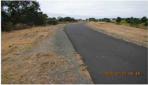
Figure 5-3: Inspection Point NLT1\_2020\_a\_0002: Drop in crown elevation.
