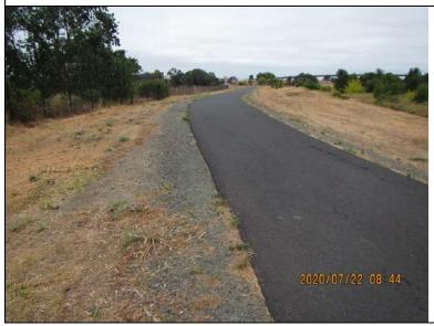
Inspect ID: NLT1\_2020\_a\_0002 Title: USACE\_CESPN\_NLT1\_2020\_a\_0002\_1.jpg Rated Item: 6. Erosion/ Bank Caving Caption: Rating: Acceptable; Remarks: Drop in crown elevation for the last 200 feet.; Action: Monitor.
